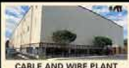
CABLE AND WIRE PLANT
