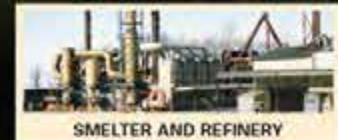
SMELTER AND REFINERY
